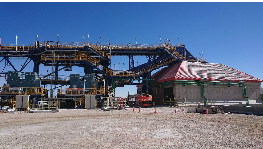
Image 12: Bunker building with material discharge from the overland conveyor OLC-01
