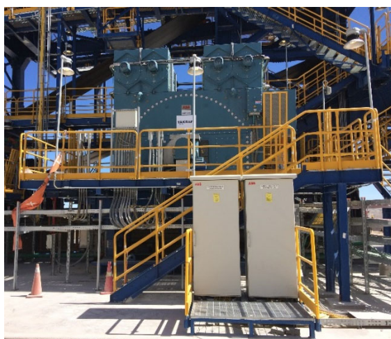
Image 4: 5 MW drive once installed
