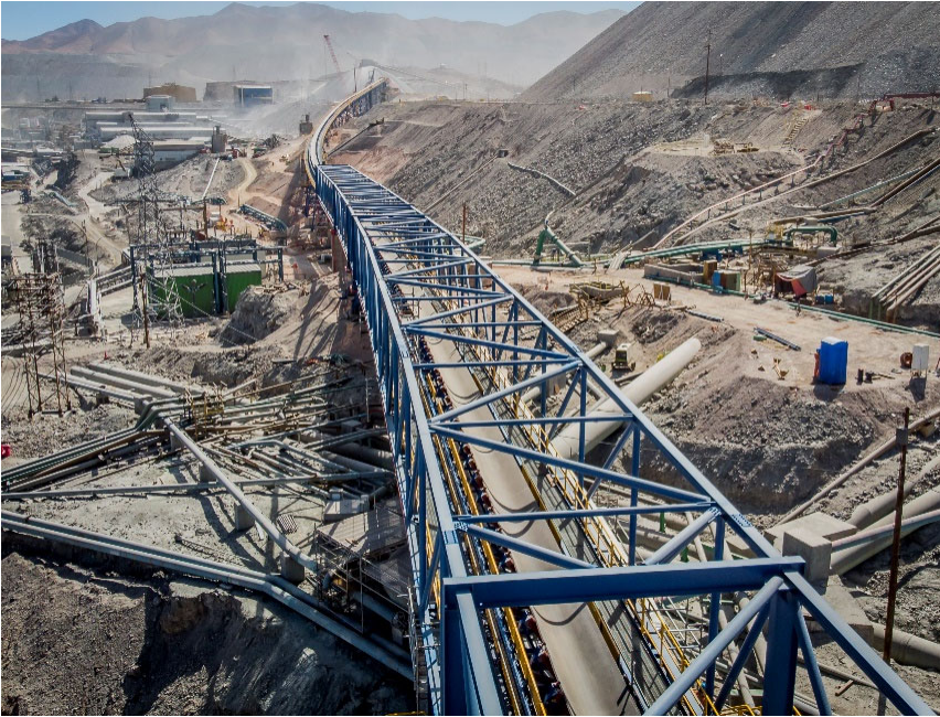
Image 9: Overland conveyor OLC-01 passing over existing infrastructure
