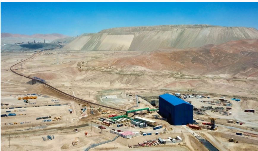
Image 8: Overland conveyor OLC-01 with feeding point in the drive house of the inclined conveyor C02 (blue building)
